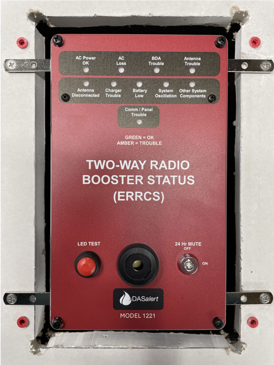
Figure 8. Mount panel into cavity with supplied # 6 flat head screws. Attach power and wiring from BDA, BBU and Fire panel
